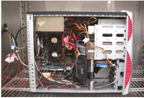
The view of the thermocouples connections.
